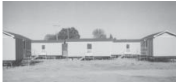
VWS built new migrant worker housing in Sonoma, California.
